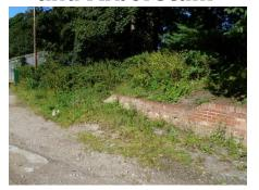
The clearance of a large amount of debris accumulated over the past 20 years has been removed revealing the continuity of the dwarf brick retaining wall and an embankment supporting the remnants of the historic path to Norton Hall walled garden.
