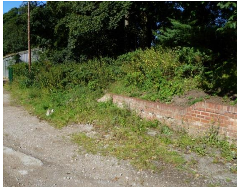
Wall before clearing embankment
