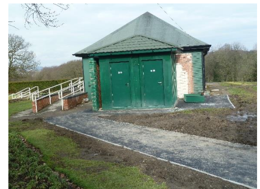
The Refurbished Toilets
