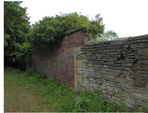
Nursery Wall - Stone to Brick
