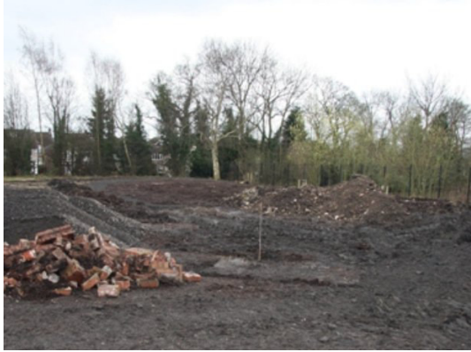
The Chantreyland Meadow landscaping in progress
