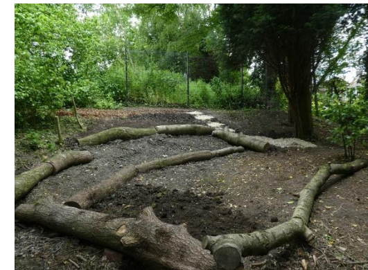
New Dell Area Construction
