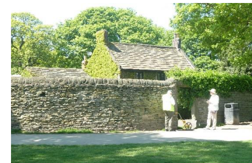
Surveying Graves Park North Wall, with Bole Hill Farm in the background, May 2019
