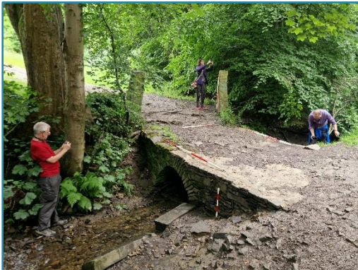
Surveying the Packhorse Bridge
